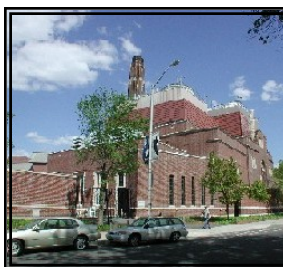
Yale is working to reduce emissions from its Central Cogeneration Power Plant.
